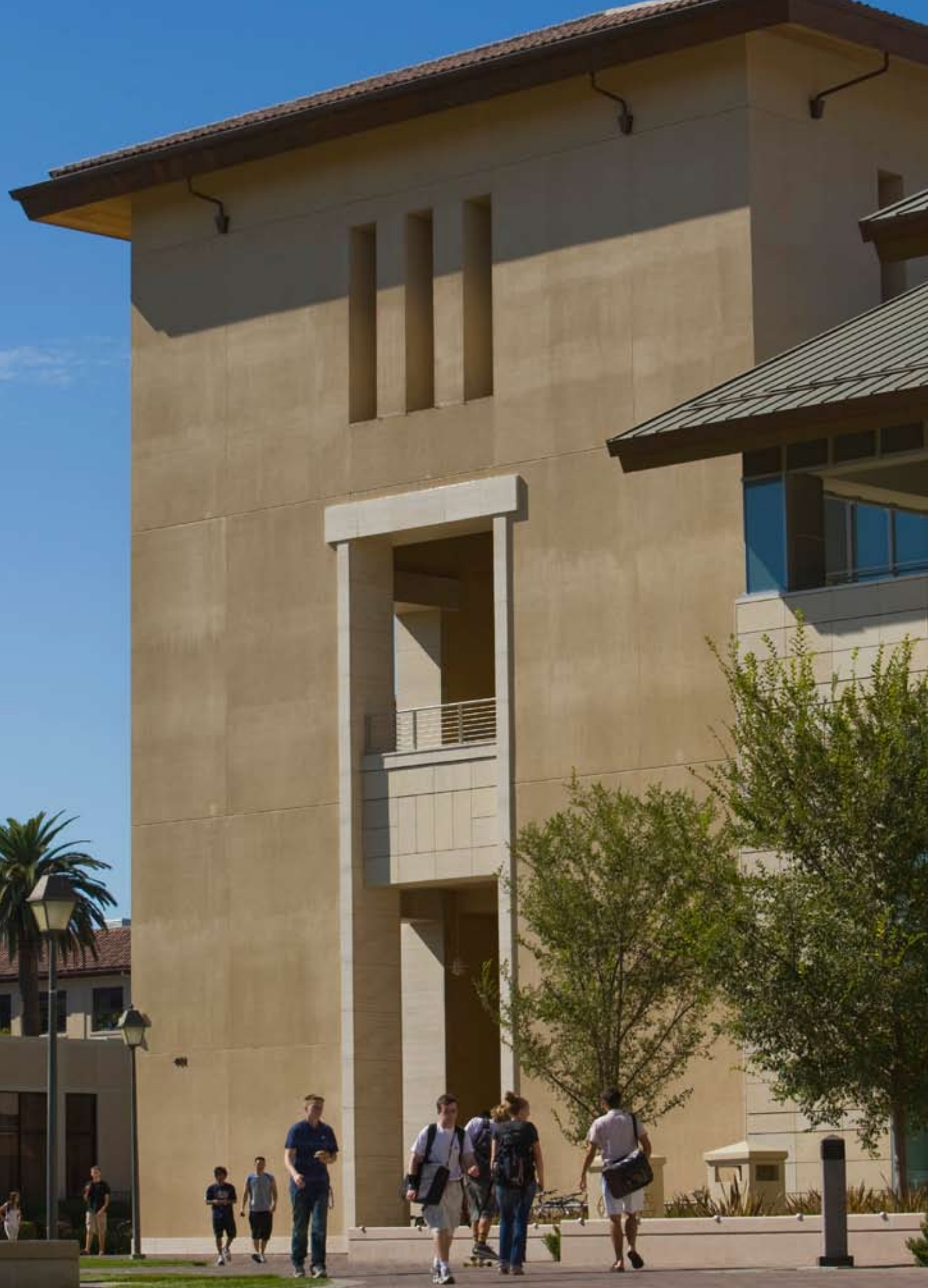
Though twice the size of the former Orradre Library building, SCU's new Harrington Learning Commons, Sobrato Technology Center, and Orradre Library use about the same amount of energy.
