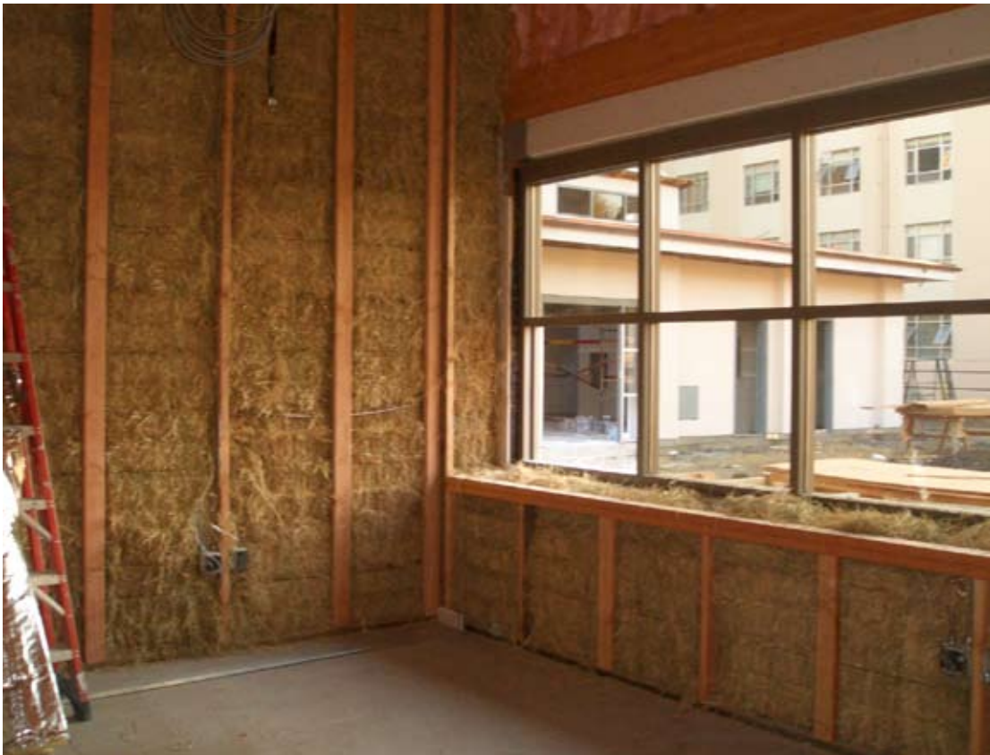
Photo courtesy of Devcon Construction
